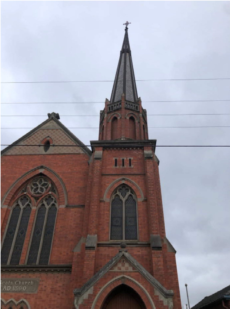
Spire with the lean to the north clearly visible
